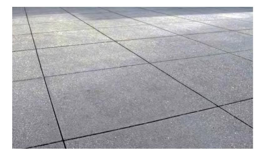
VEHICULAR COLORED SAWCUT CONCRETE PAVING
