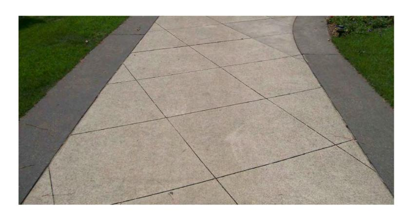
PEDESTRIAN COLORED SAWCUT CONCRETE PAVING
